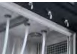
Fig. 6: Guide rail for plexi divider. Alternatively, a fixation with pins and loops is used.
